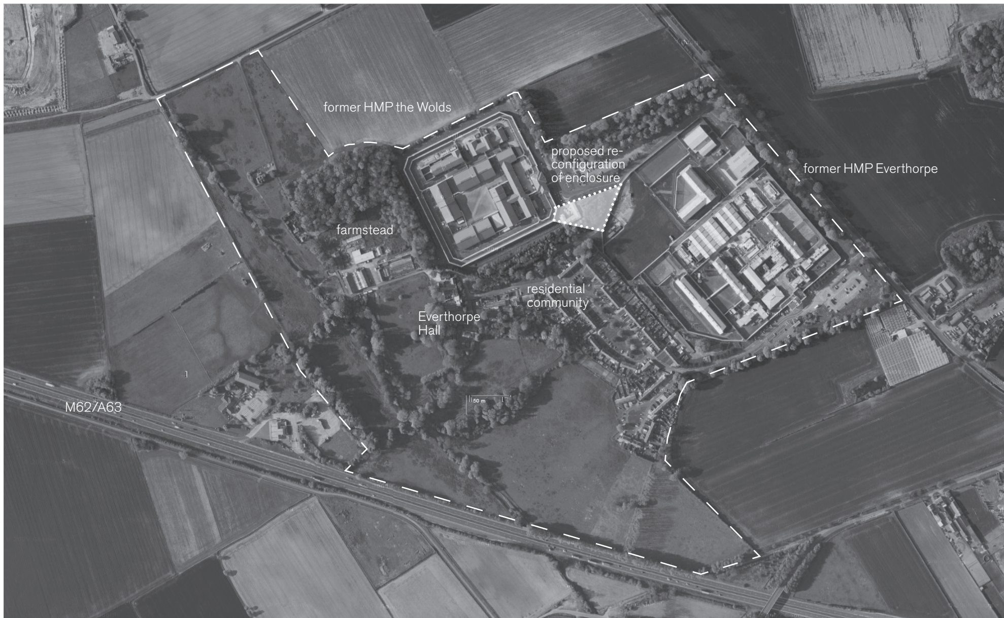
Aerial photo of the HMP Humber site ©2013 DigitalGlobe, Getmapping plc, Infoterra Ltd & Bluesky
